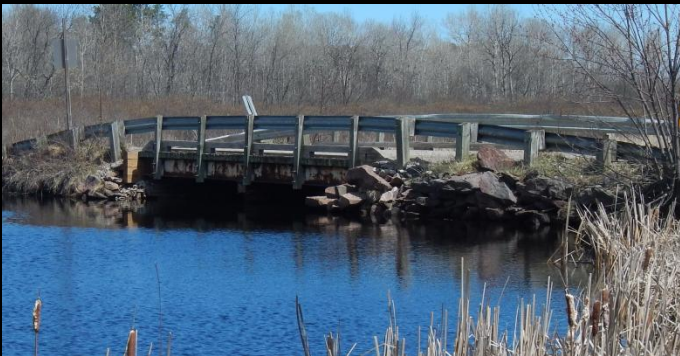
Photo 1: Upstream face of existing 9.6m span stringer bridge looking North-easterly.
