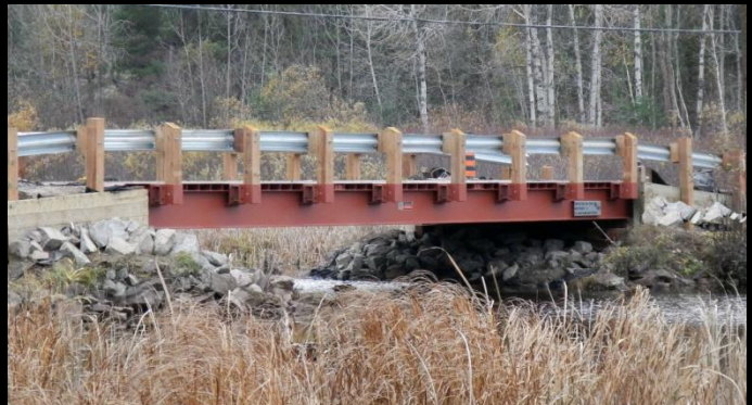
Photo 4: Downstream face of new 15.2m span Lessard Modular bridge. Pile cap removed as part of old bridge removal/new bridge installation.
